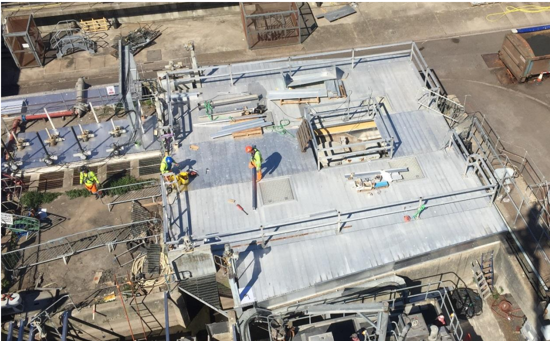
Installation of odour control aluminium flat deck system at Portswood WWTW
